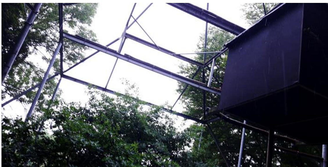
Picture 3: The aviary is made with round iron pillars and rectangular iron crossbars.
