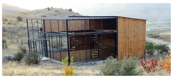
Perches are installed throughout the aviary, at least 60cm away from the mesh, and at the same level as the platform following the EEP recommendations but only 13cm wide, not giving birds enough stability by matting. Further a spiral step has been installed in front of each platform but with only 50cm large and 13cm wide steps, and with 25cm step height, making the climb to the platform difficult without breaking feathers.
