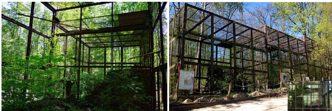
Picture 3-5. Aviaries are built on an iron structure divided in iron pillars and beams each 2m and covered with wire mesh.
