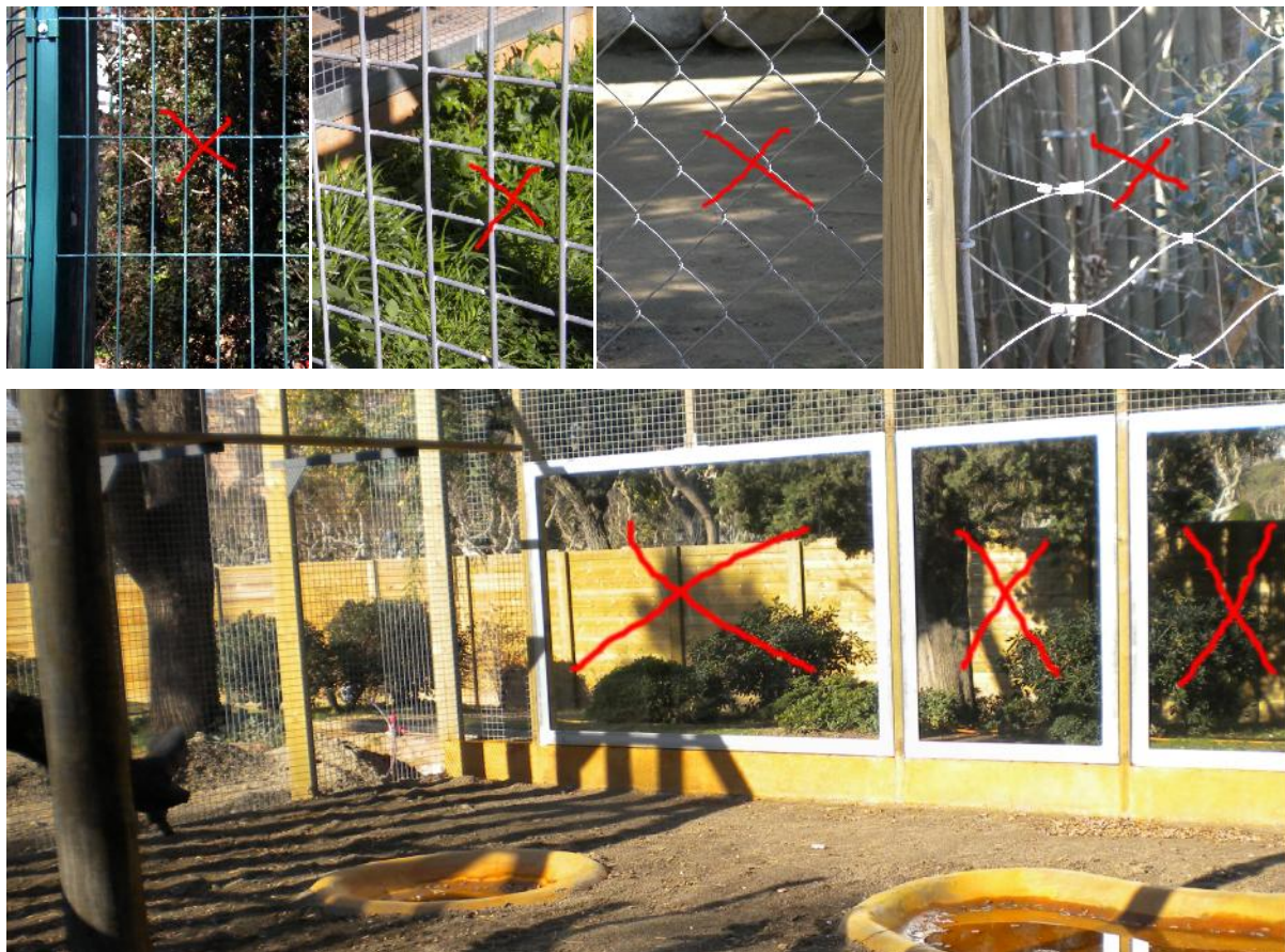
Above left: two examples of hard mesh. Above right: two examples of adequate soft mesh. However, the mesh size is larger than 4 x 4cm and thus does not prevent entry of small predators, such as martens ( Martes sp. ) and genets ( Genetta genetta ) to the aviary. Below: glass enclosure, which can cause deaths through collision.
