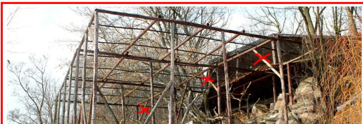
There should be no reinforcement structures inside the aviary. Frightened birds fly “blind”: they do not look where they are going, because they are looking in the direction of the perceived danger.
