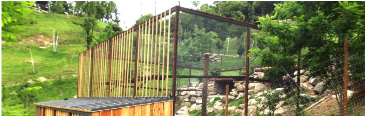
Wooden laths (4cm wide by 2cm thick) every 20 cm to prevent injuries caused by birds flying into the side of the aviary (Bearded Vulture aviary at the Parc Animalier des Pyrénées, France).
